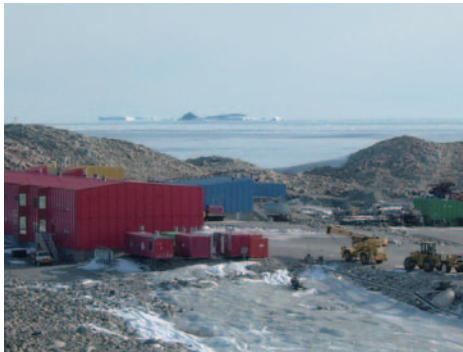
Photo 15 ケーシー基地の建物 Photo 15 Buildings of Casey Station.
