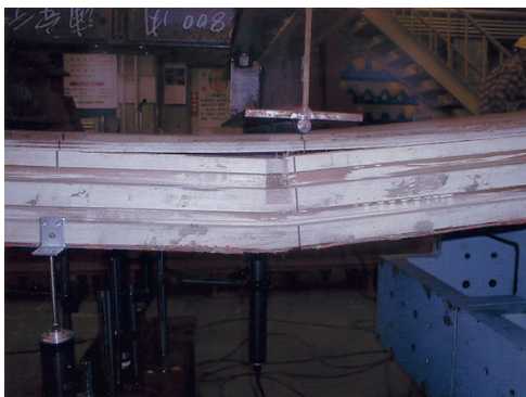
図 20 床パネル圧縮側合板の剥離 Fig. 20. Separating fracture of the surface plywood plate of floor panels.
