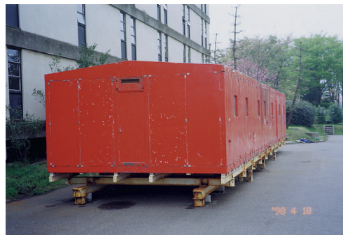
図10 居住棟の復元工事4 復元工事完了 Fig. 10. Reconstruction of the living hut. Final phase: Completion.
