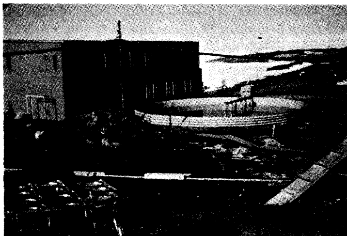
Fig. 9. Outdoor 100-kl water tank set near the new engine room.
