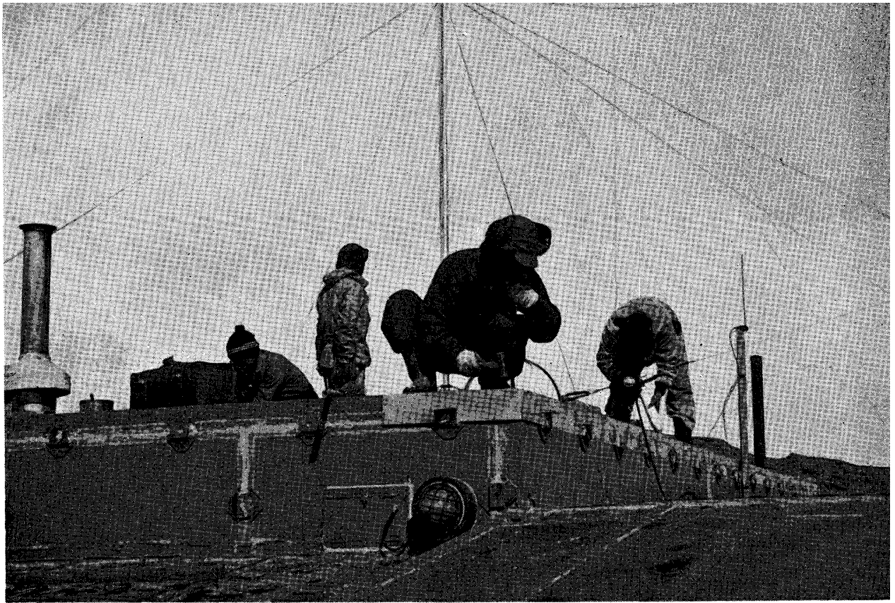
Repairing and strengthening huts of the station.
