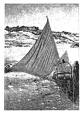
Fig. 6. The sail of dog sledge, which was made of duralumin pipe, nylon sheet and nylon rope, have a main pole, not stood vertical for the sake of getting a wide range of vision in front. It weighs only 4.8 kg altogether. The sledge in this figure is of rattan. There are two magnetic compasses in rear of sledge and in head respectively.
