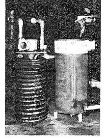
Fig. 42. Heat-exchanger for recovering the engine exhaust gas energy (not yet insulated and in the state of overhauled).
