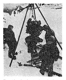
Fig. 18. Steel tripod and chainblock lifting up a gasoline engine at the Syowa Base.
