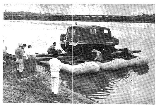
rubber boat was used only for boating excursions in the Antarctic in 1958. Total length : 6.180 mTotal beam : 1.680 mDia. of air-chamber : 0.560 mWeight : 85 kgCollapsed volume :  $0.6 \times 0.6 \times 1.5 \text{ m}$
