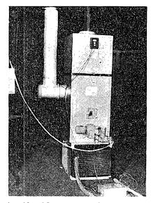
Fig. 39. New system for recovery of exhaust-gas heat of 40 IP Diesel engines driving 20 KVA electric generators (A heat-exchanger was placed at the inlet of room air to the warm-air heating furnace).
