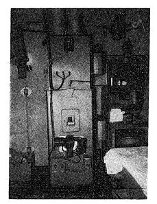
Fig. 32. Pot type warm-air heating furnace MHF-40 D type set in a living-room of the Syowa Base (prepared by Minorikawa Factory).
