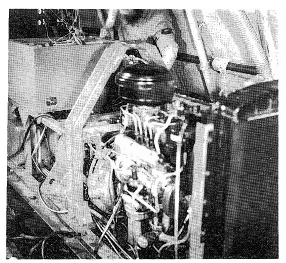
Photo. 10. Inside view of engine room and a 20 KVA Diesel electric generator.
