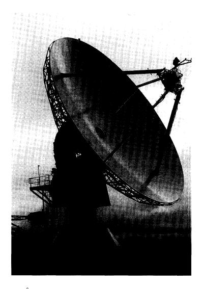
Fig. 1. The Ny-Ålesund VLBI antenna. A 20 m diameter dish with the S/X receiver in the primary focus.
