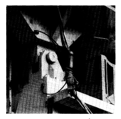
Fig. 3. Particular of the elevation axis of the VLBI antenna in Ny-Ålesund where the pin (marker 50) has been set up. One of the Leica tape target used for testing the marker 50, is also visible. At the symmetric opposite side the marker 51 has been set up in the same way.
