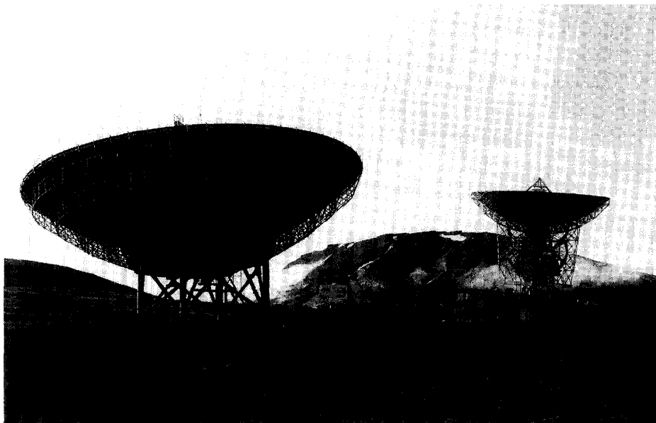
Fig. 1. The EISCAT Svalbard Radar (ESR) with the 32-m steerable dish in the background and the 42-m fixed dish in the foreground (September 1999).
