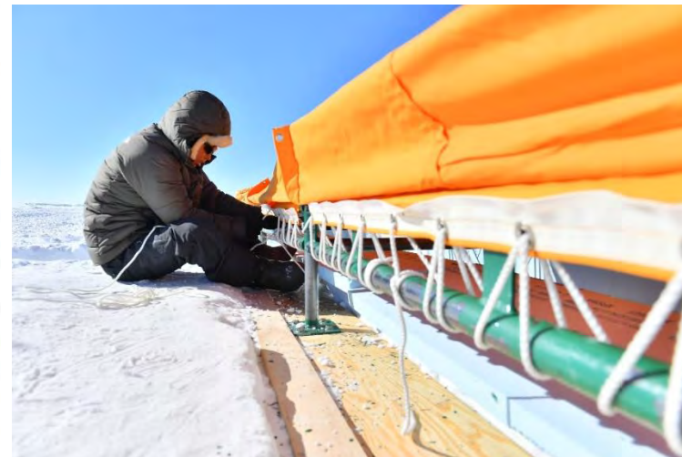
屋根膜の取付
