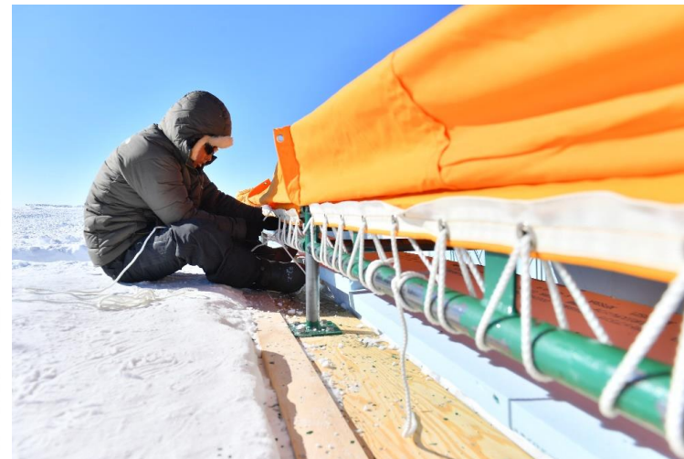
屋根膜の取付
