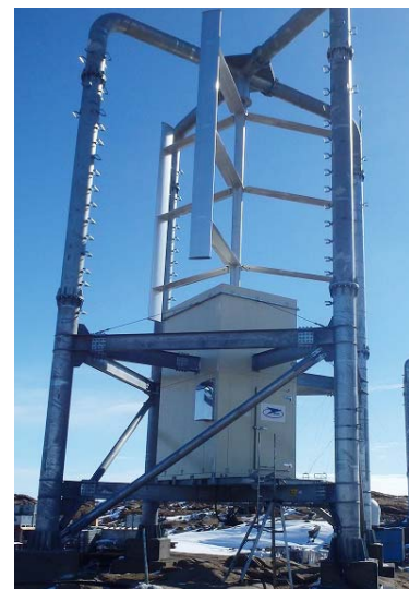
20kw wind turbine installed at Syowa Station
