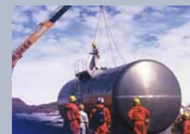
Installation of fuel tank
