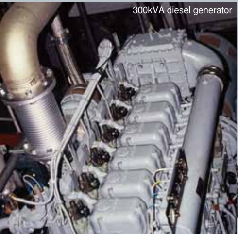
300kVA diesel generator
