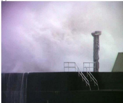
(B) Fig. 2. Two dummy lighthouses set up on the north breakwater of Hamamasu harbor. (A) Spray jet generated by the breakwater, (B) Impinging of spray jet and green water.
