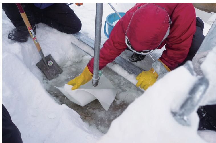
図 13 防油堤の底に溜まった油の回収 Fig. 13. Recovery of spilled oil at the bottom of the reservoir.
