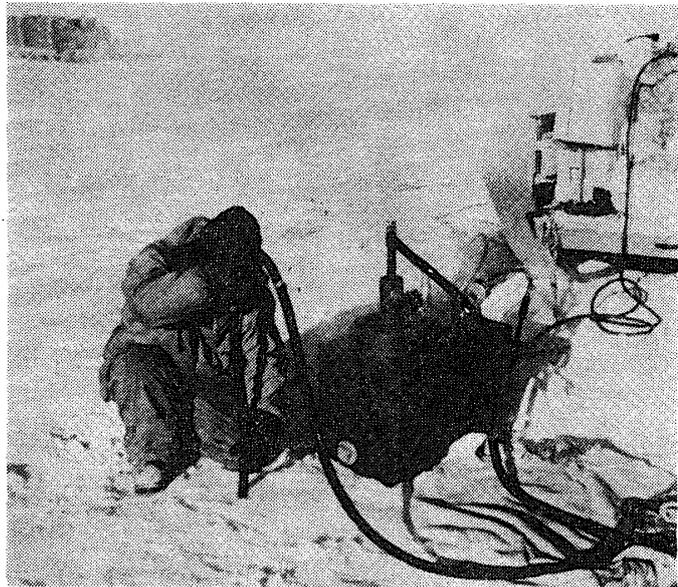
Fig. 2. Drilling with the steam drill on the snow at Mizuho Plateau, East Antarctica. A propane tank is placed on the sledge.
