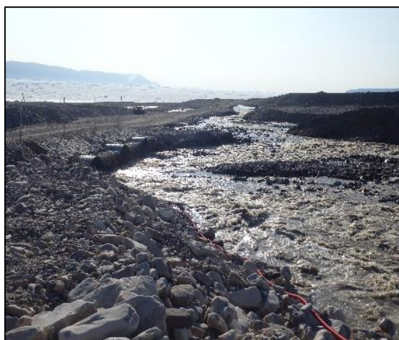
Figure 1. The flood event on 17 July 2022.
