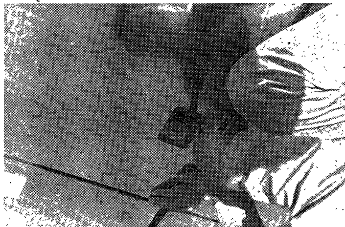
Photo. 1. For the connection of two panels, each bolt is easily inserted and screwed through a hole opening inside a hollow on each panel.
