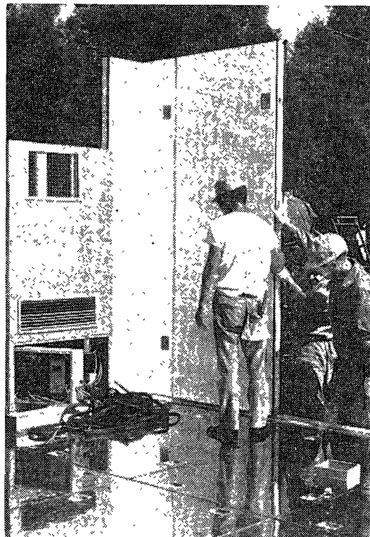
Photo. 6. A wall panel is connected with the corner panel.
