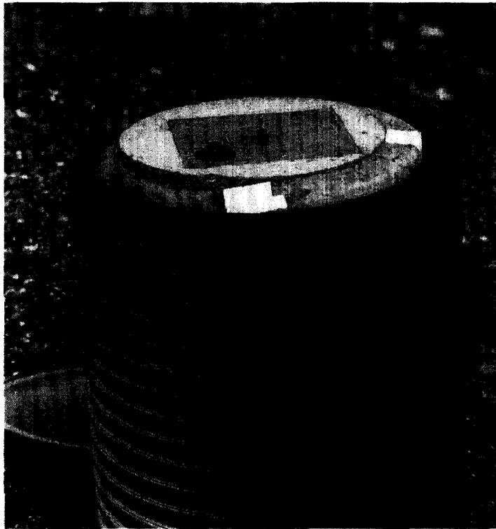
*Fig. 6. One of the pillars of the control network around the VLBI antenna of Ny-Ålesund. It is visible the metal plate on the top of the pillar with the Wild central screw for horizontal reference and the ex-centric levelling bolt for height reference. All the pillars are equipped in the same way.*
